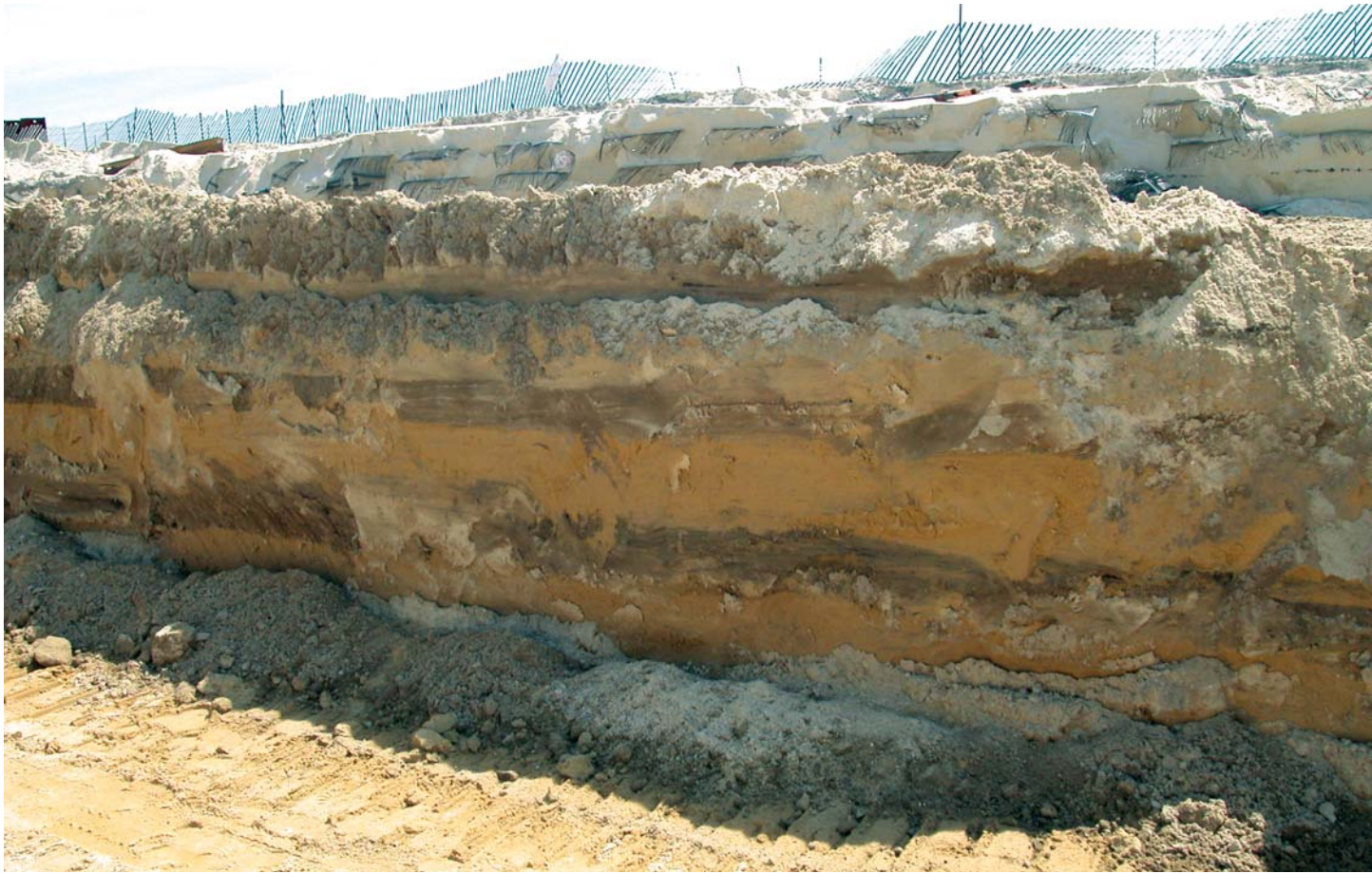
FIGURE 1 Apparent cohesion allows for unreinforced vertical cut in medium-fine sand.
